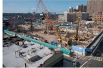
Building site security
