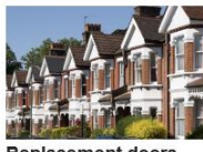
Replacement doors and windows
